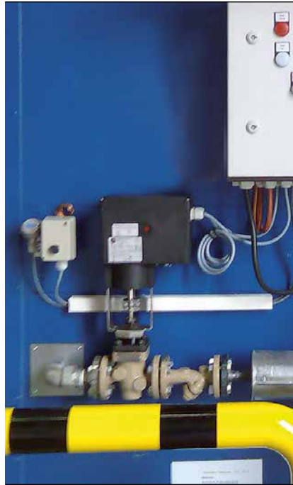
Steam heating with temperature regulation, electrical
