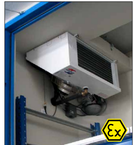
Split cooling unit (inside view) in explosion proof design
