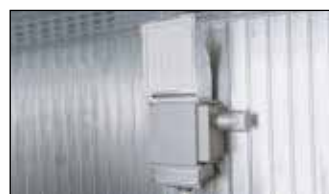
Heating fan for active, targeted convection in larger walk-in hazardous materials stores.
