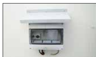
Sub-distribution unit (e.g. when sockets are used)
