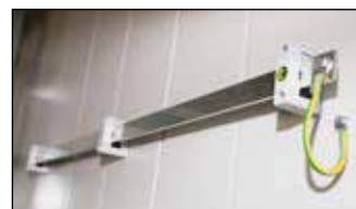
Earthing rails inside the technical room system
