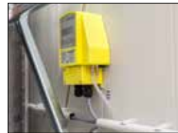
Air extraction monitoring for air exchange > 2.0/h
