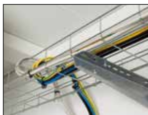
Cable duct for clean routing of internal wiring
