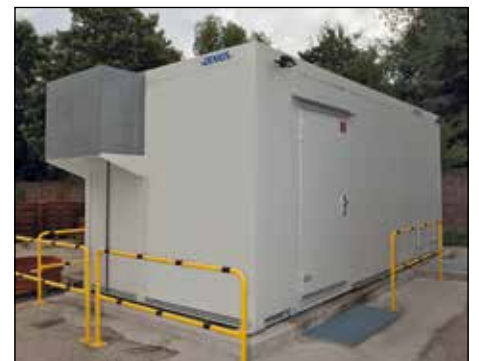
Impact protection barriers offer additional protection for the IT Container
