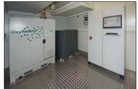
View into the technical room: Oxygen reduction equipment, UPS, monitoring
