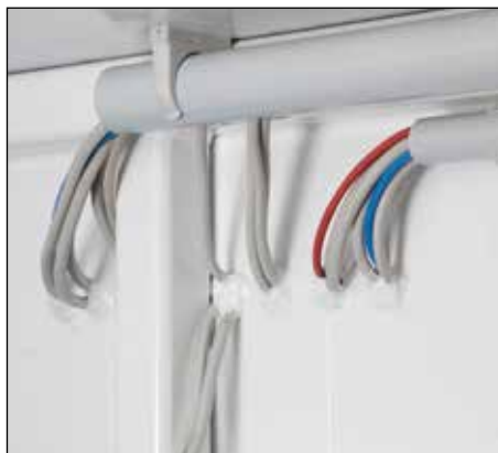
Fire protected break-through points for cables in a side wall
