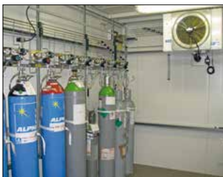
Housing for technical gases in a climate controlled safety room with fire protection
