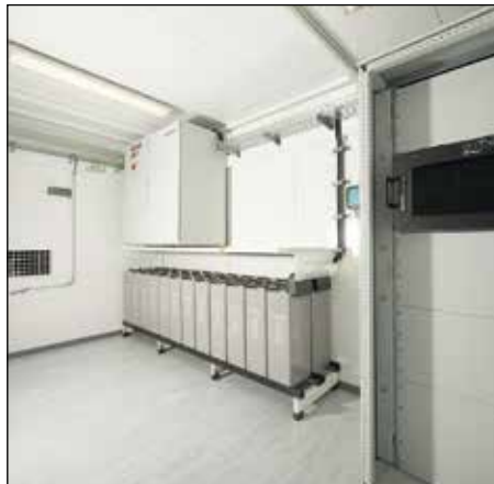
View into the technical room with fuel cells and corresponding storage media
