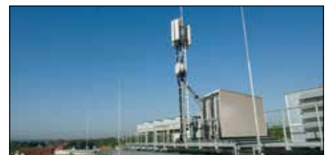
Radio centre with technical / safety room on the flat roof of an administration building
