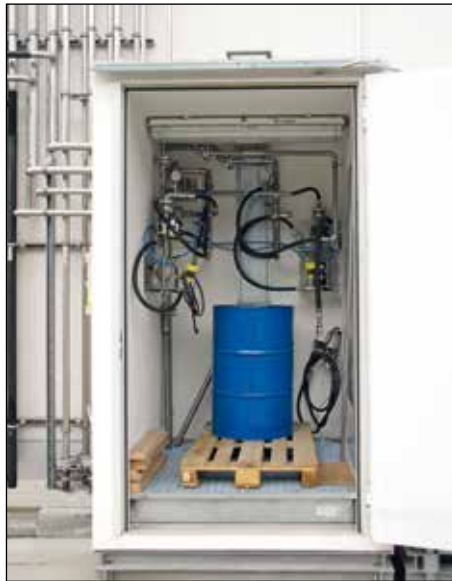
Fuel metering for engine test rigs -internal view
