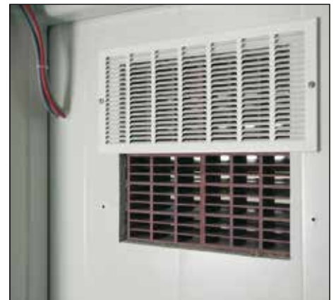
Ventilation brick with safety melt feature
