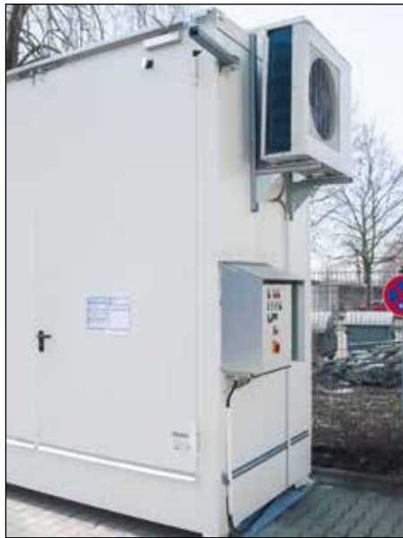
Specific temperature control for a battery storage container
