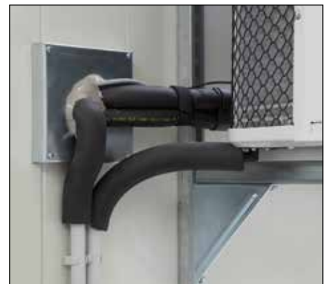
Fire protected break-through points for pipework in a side wall
