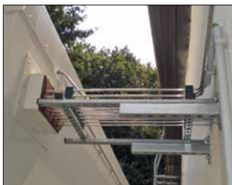
Firestop brick and piping into building
