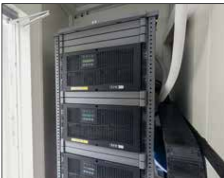
The UPS is separated from the IT technology – in a second fire area
