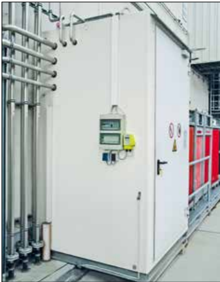
Fuel metering in safety room with fire protection
