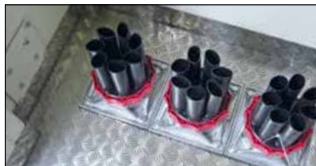
➡ Left hand photo: Floor break-through points with fire and rodent protection, gas and water-tight
