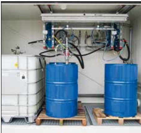
Active, fire-rated storage of flammable substances
