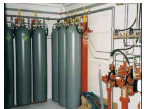
CO 2 extinguishing gas cylinders, ready connected
