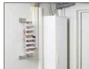
Switch cabinet and data transfer point
