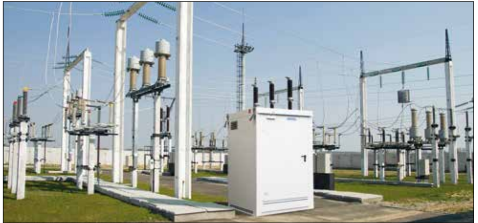
Substation with decentralised technical / safety room
