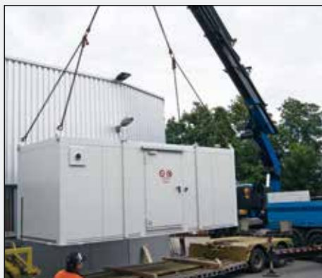
Unloading with a truck-mounted crane, installation on the prepared foundation
