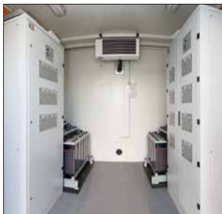
View into the uninterruptible power supply (UPS) in the container
