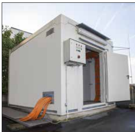
F90 fire-rated container, cable routing in the double floor
