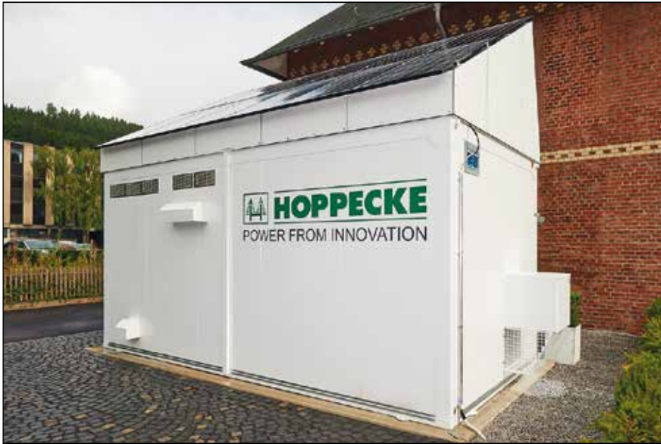
In addition to fuel cells, photovoltaic equipment was also sited on the container roof to provide a source of energy
