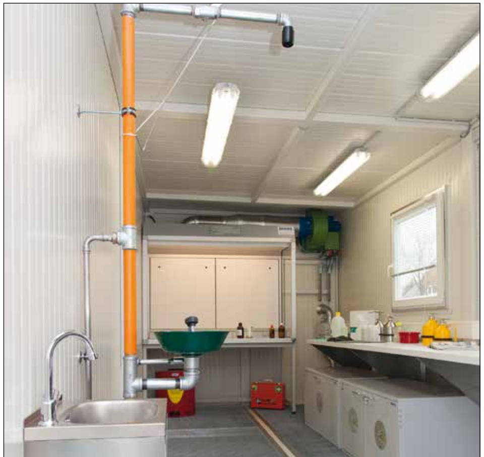
Sampling / analysis room with air technology workplace and emergency shower. Additional safety is offered by fire-rated underbench cabinets for retained samples
