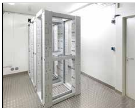
Passive IT infrastructure - ready for customer to fit out
