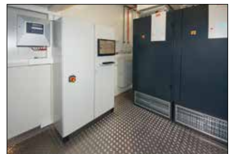
Also in the technical room: redundant climate control equipment
