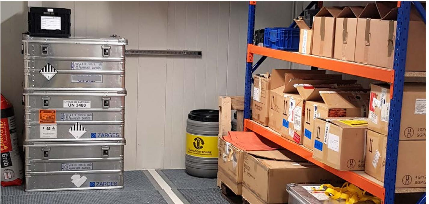
The entire technical room system has F 90 (REI 90) fire protection with an IBS classification report (Institut für Brandschutztechnik und Sicherheitsforschung - German Institute for Fire Protection Technology and Safety Research). In order to accommodate the large drive batteries weighing up to 700 kg and the small battery cells in a practicable way in one technical room system, the room is divided into two sections: one accessible and one that can be loaded with a forklift truck.
