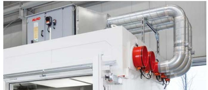
Fire protection flaps for ventilation system
